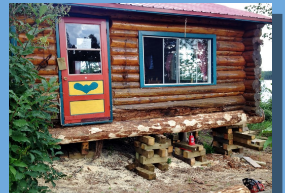
First log is in place!
