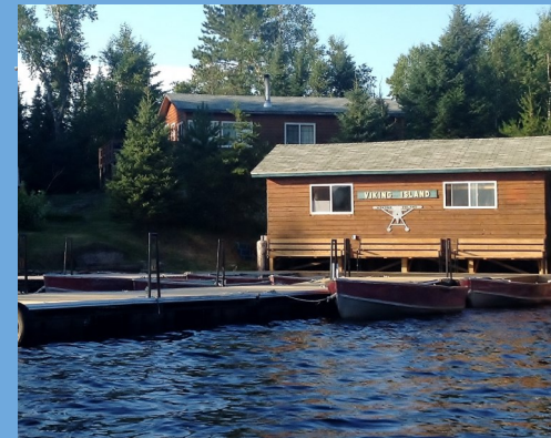
Stage 1 of the docks finished!
