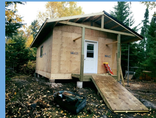
New laundry and shower house during construction
