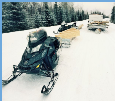
Hauling in roof trusses for the laundry/shower house
