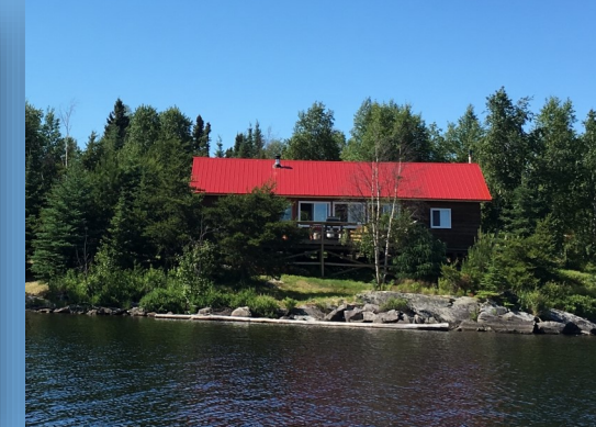
New roof & supports on the Fireside
